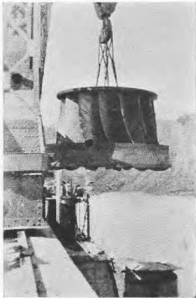
Placing water wheel of Unit No. 2 at Mitchell Dam
